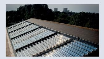
The installation generates 44,100 kWh/year of annual thermal output and 3,487 kWh/year, resulting in 4981 kg of carbon saving each year.
